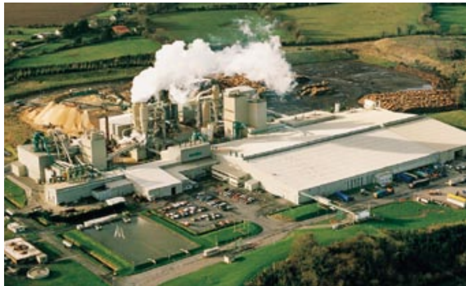
Aerial view of the Medite plant
